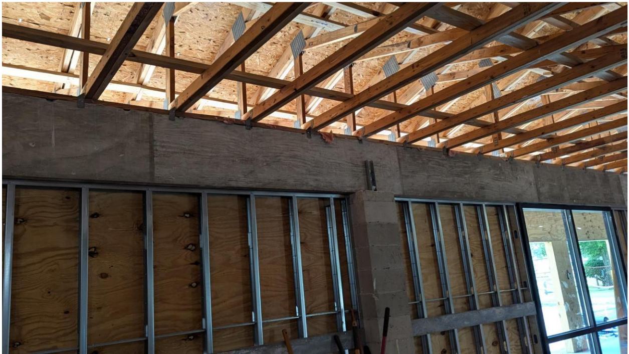
Rafter Clips – North Wall (Typ)
